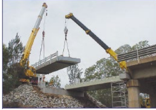
Figure 2.5: First Composite Bridge in Australia (Jonathaan DePlanche, 2003)
