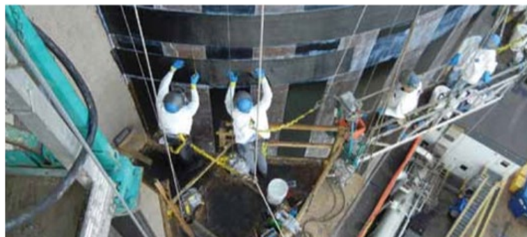
Figure 1.7: Application of FRP Materials for Strengthening Purposes (Structure Magazine)
