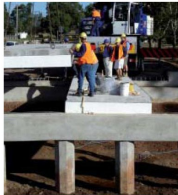
Figure 2.6: Construction of Taromeo Creek Bridge (Queensland Department of Main Roads 2005)
