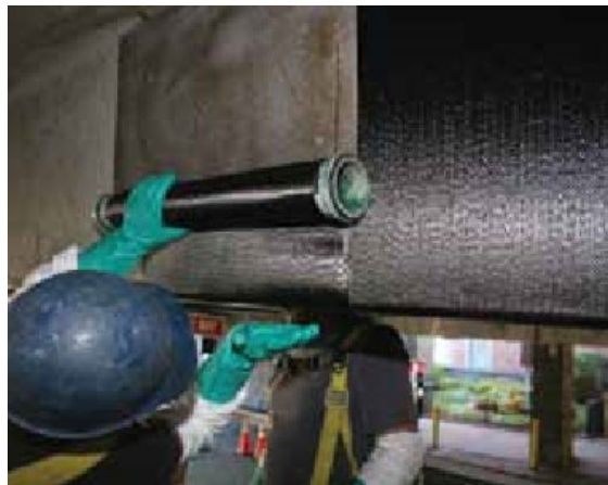
Figure 1.3: FRP Wrapping Around Existing Beams (Structure Magazine)
